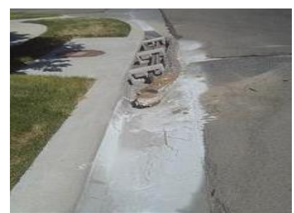
Concrete, mortar rinse water
